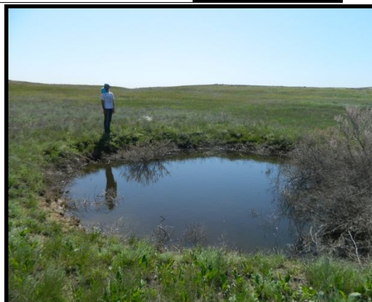
Figure 9 - Failure at Gorky Lake in 2012. (Photo by I.V. Golovachev)
