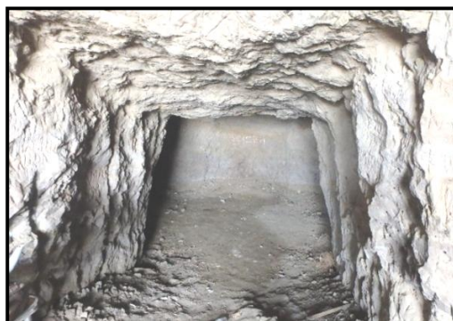
Fig.9. View inside the mine (photo by I.V. Golovachev)
